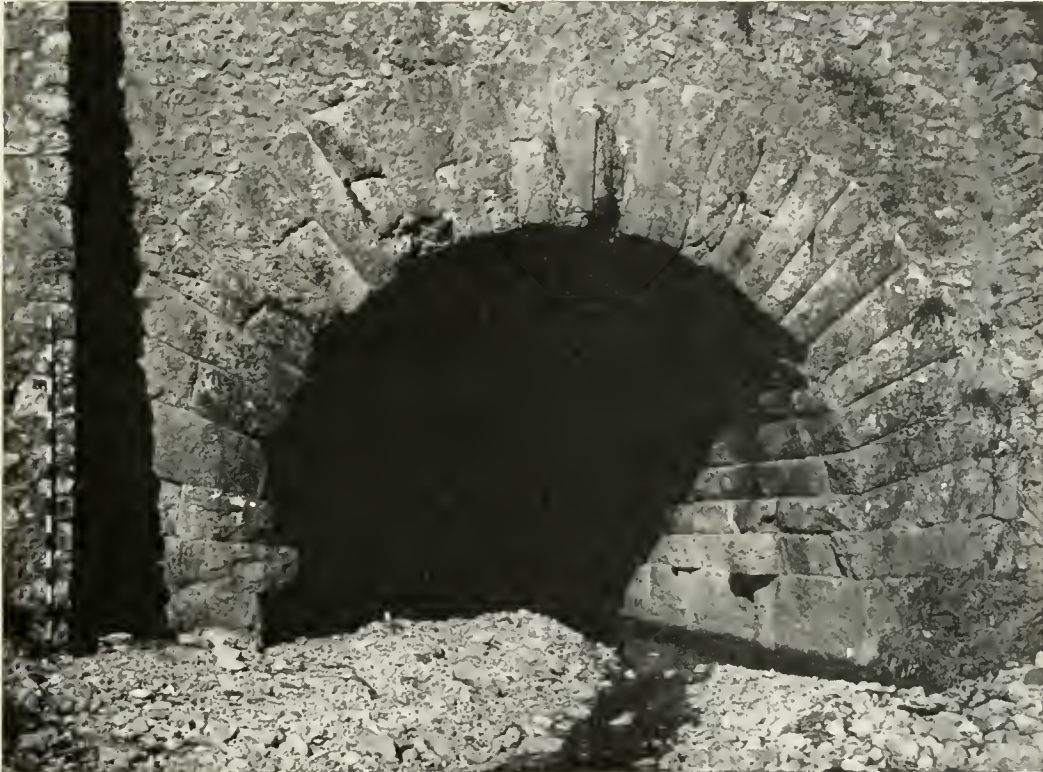
FIGURE 1. —POSTE DI SAN GIORGIO, VIEWED FROM THE EAST Only the arch of travertine is Roman
